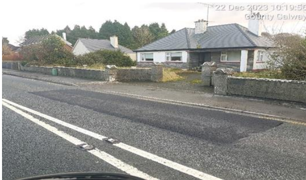
AFTER ROAD REPAIRS N83 DUNMORE
