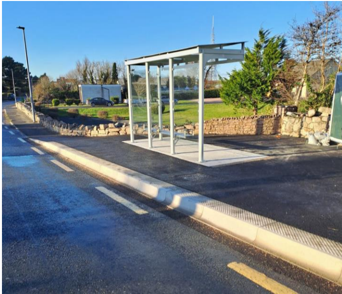
NEWLY INSTALLED BUS SHELTER CASLA
