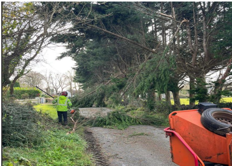
STORM DEBI TREE REMOVAL
