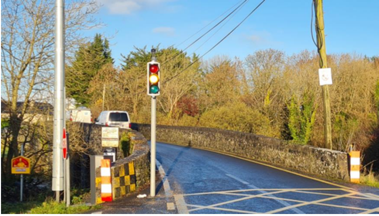
CREGMORE BRIDGE LIGHTS REPAIR
