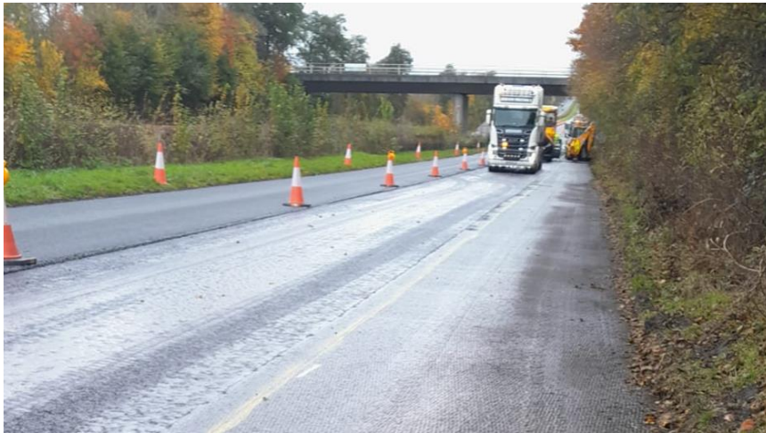
R446 DUAL CARRIAGEWAY WORKS – COMPLETE
