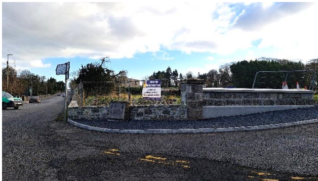
CIS SCHEME AT DÚN ÍDE ESTATE ENTRANCE, BALLINASLOE R348 - SIGHTLINE SAFETY WORKS COMPLETE DECEMBER 2023
