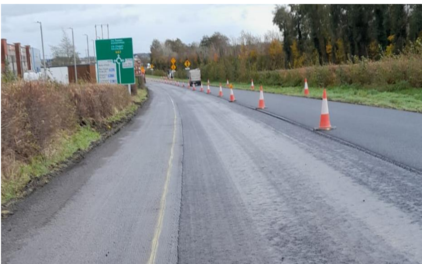
R446 DUAL CARRIAGEWAY WORKS – COMPLETE
