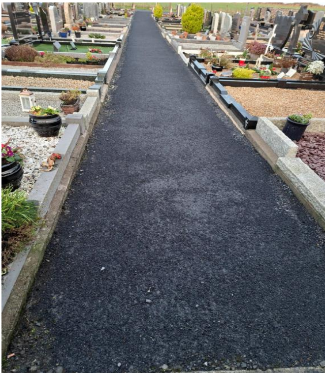
CEMETERY FOOTPATH UPGRADE WORKS – RENVILLE
